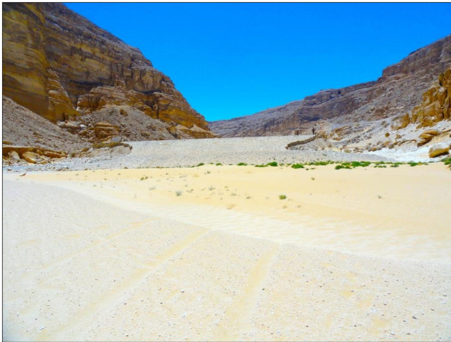
Figure 5. There is a partial collapse of the right shoulder with a length of about 20 m, as well as a collapse of 50 m in the left shoulder. Also, some traces of overtopping
