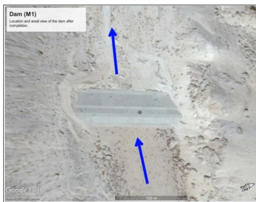
Figure 3. Satellite view of the dam before failure
