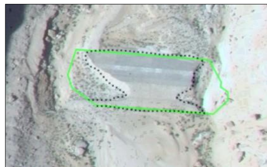
Figure 4. the dam after failure. outline of the dam (green line). boundaries of the collapse (black dotted line)
